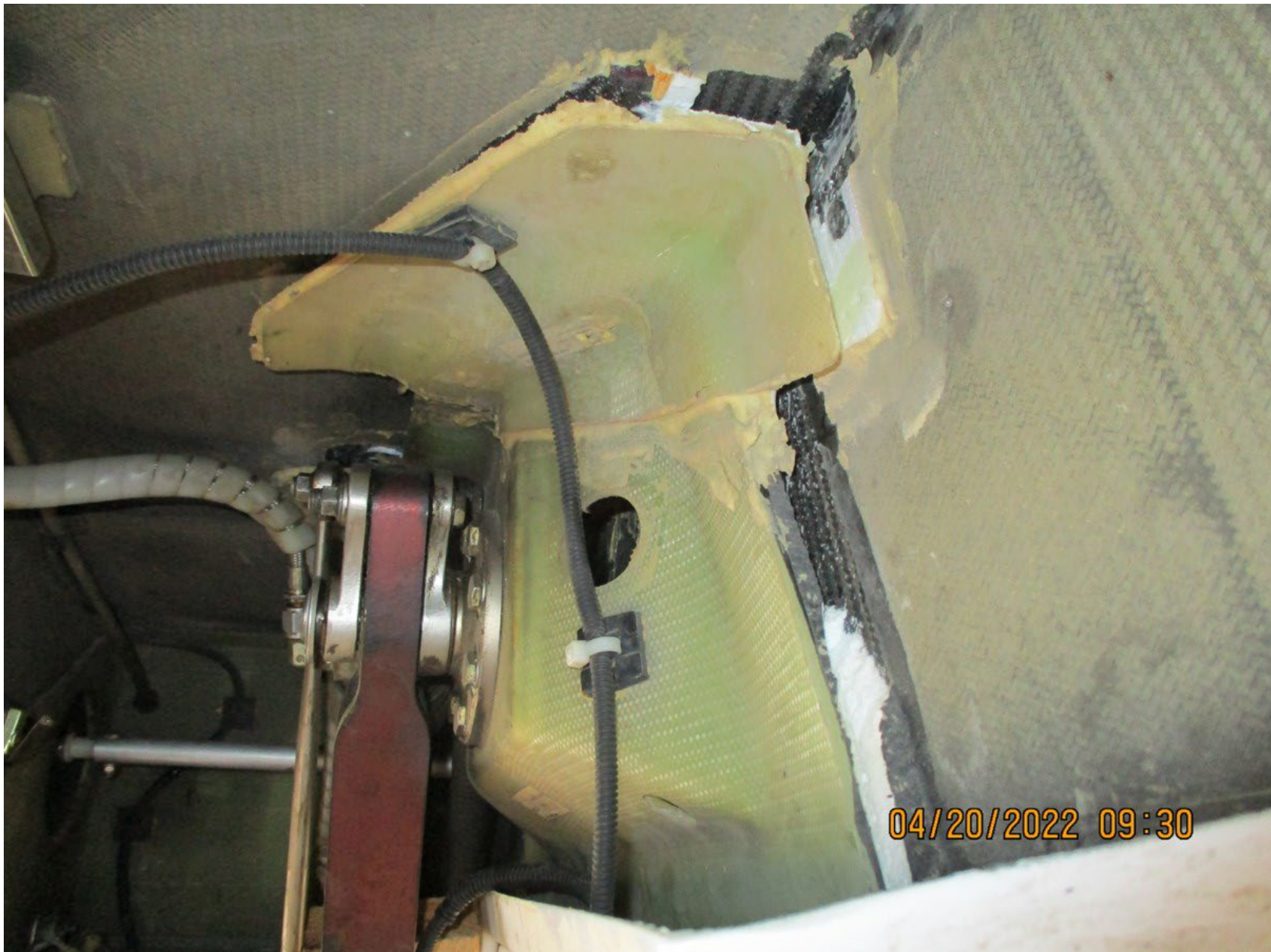
Photo 2 – Image of the landing gear support assembly. Photo courtesy of the operator.
