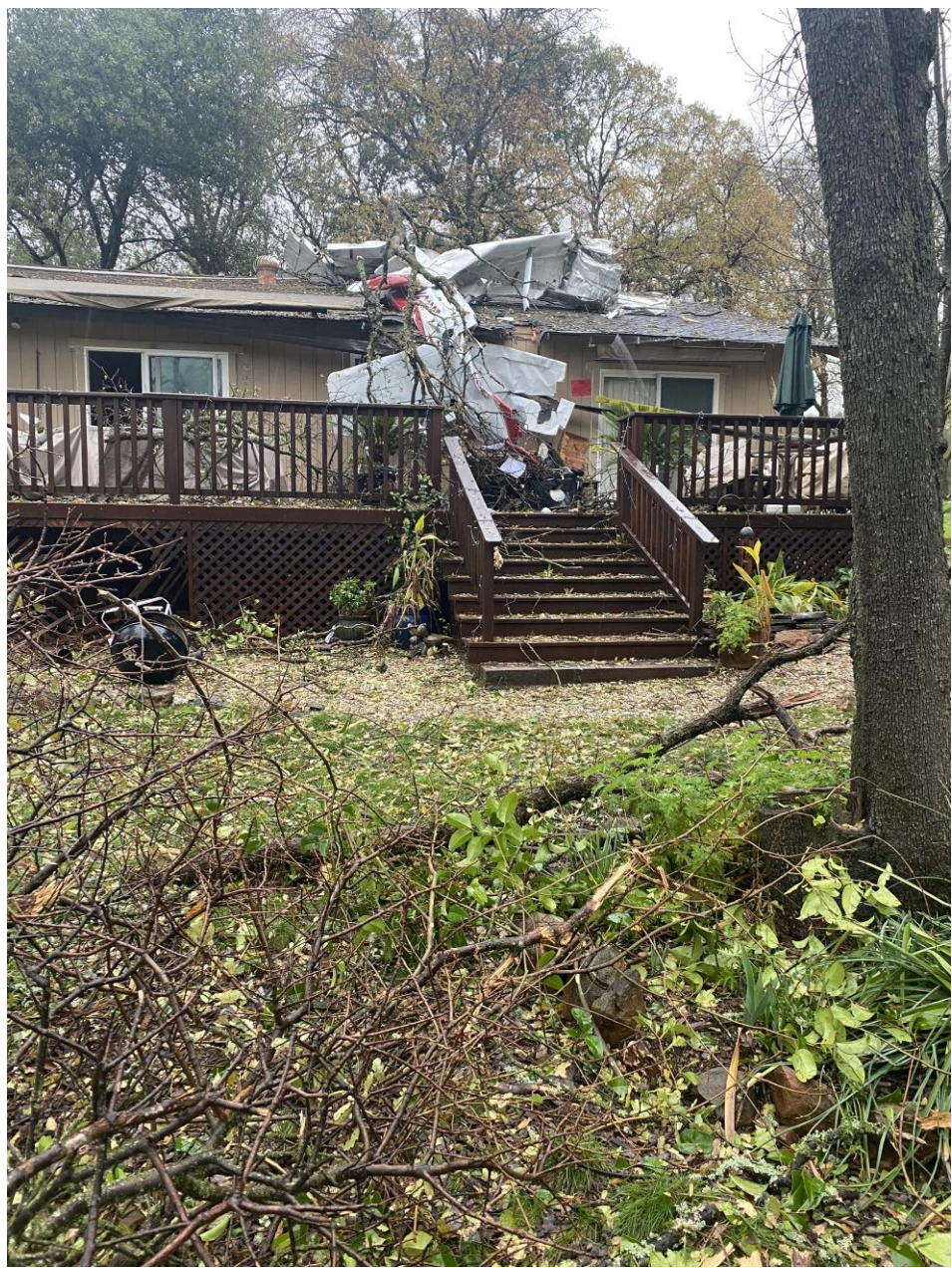
Photo 1 – View of damaged airplane coming to rest on a roof top (courtesy of FAA)
