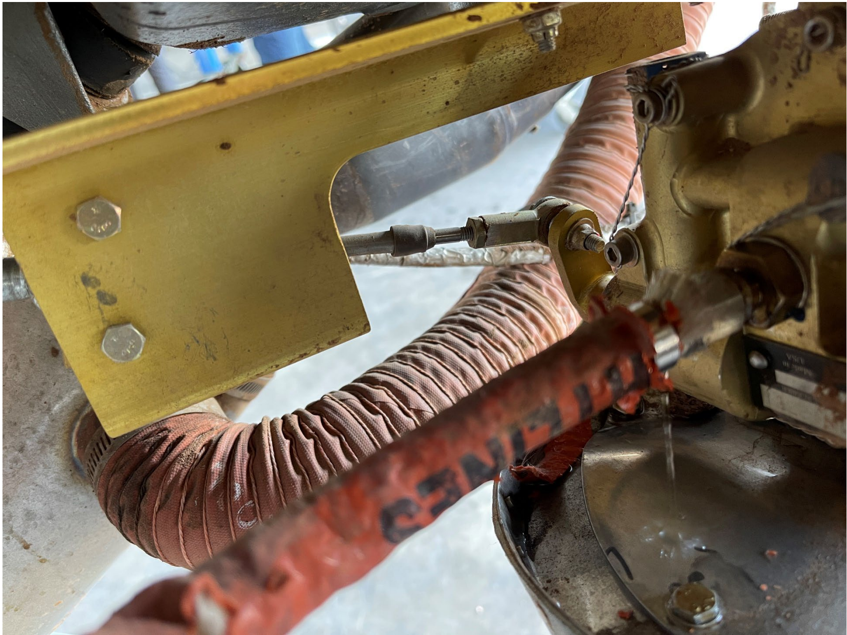
Photo 4 - View of the outlet fuel line at the fuel servo (with fuel leaking from the fitting)
