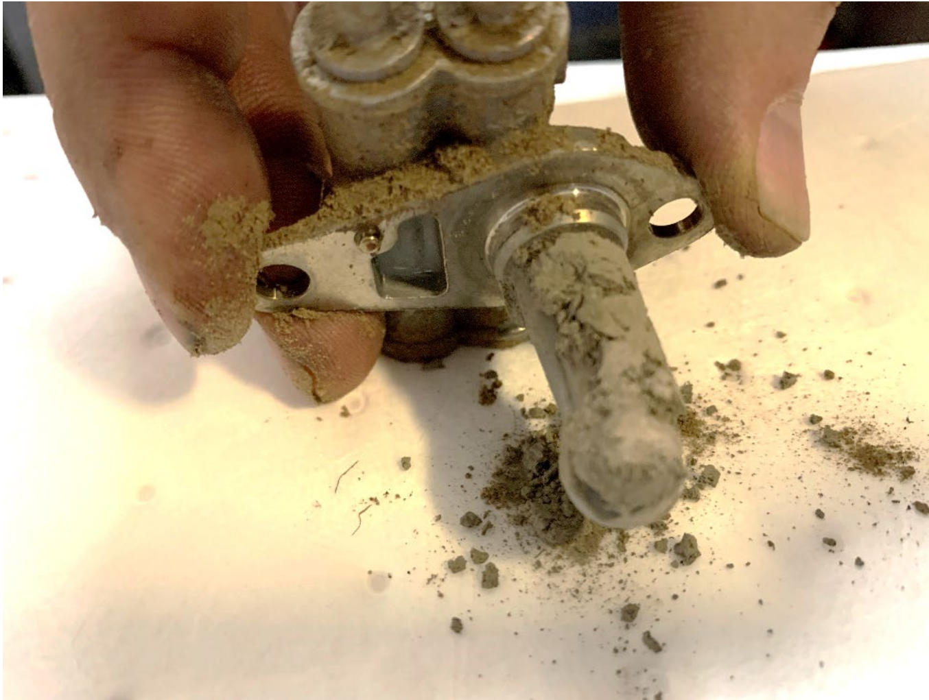
Photograph 5 - View of a fuel nozzle removed packed with environmental debris
