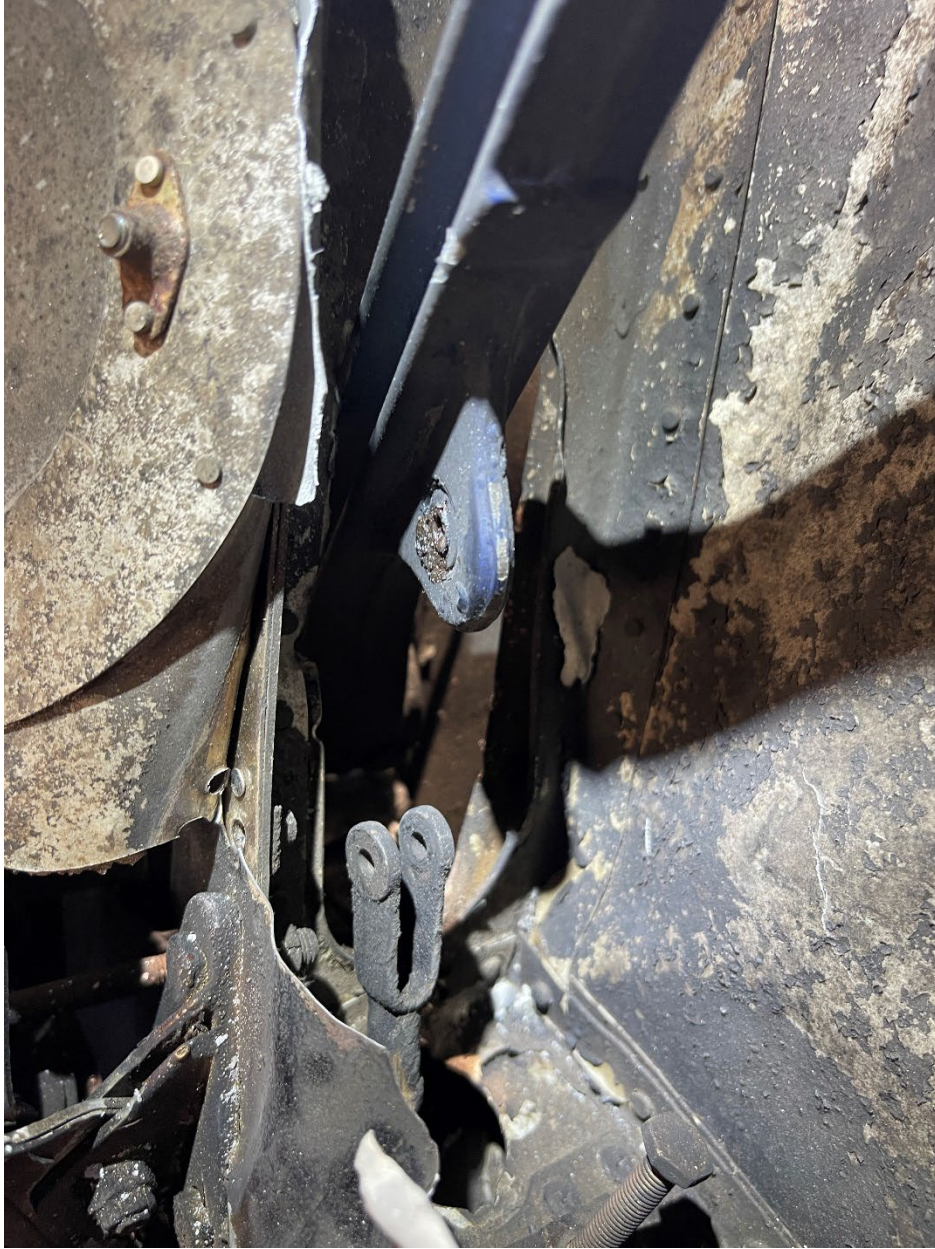
Figure 8: View of the separated control rod (balance weight to elevator).
