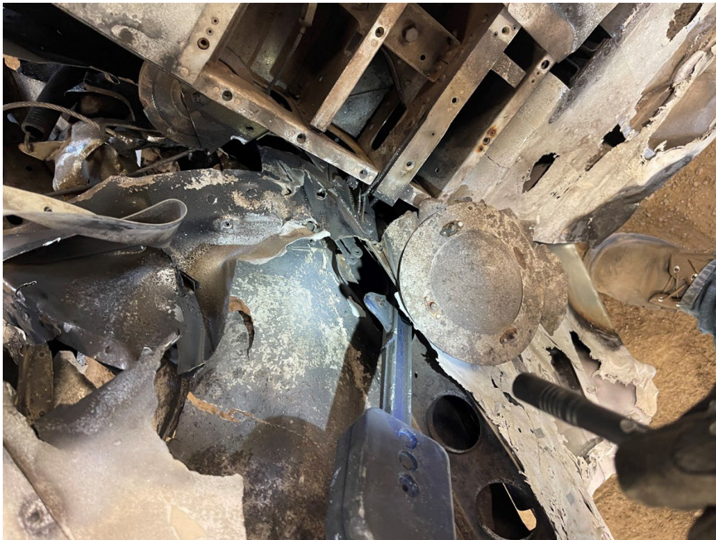
Figure 7: View of the separated control rod (balance weight to elevator).
