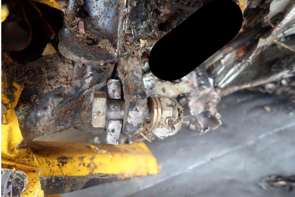
Figure 27 – Right wing strut lower fuselage fitting
