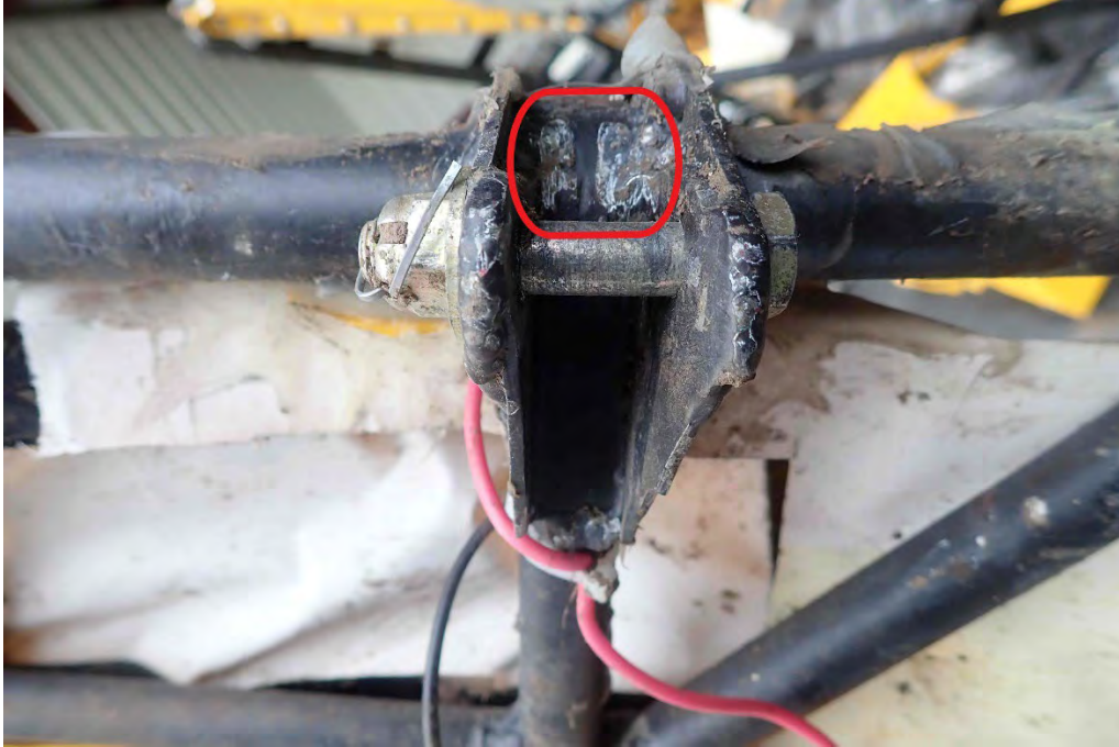
Figure 37 - Forward right fuselage wing cap assembly with notches
