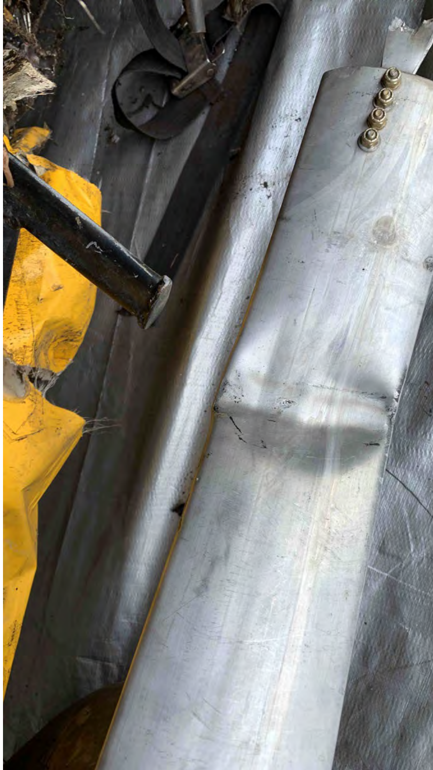
Figure 30 - Right wing strut and contact area with step
