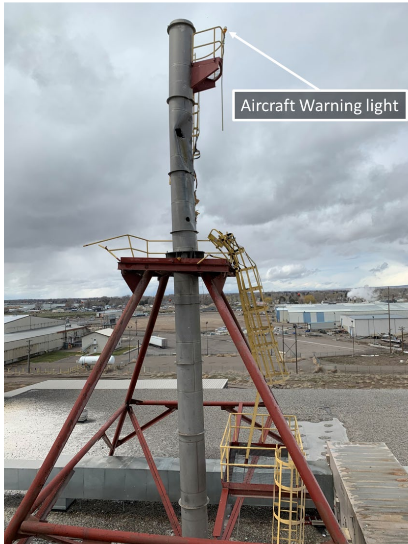
Figure 7. Postaccident photo of the agglomerate stack that the airplane struck.
