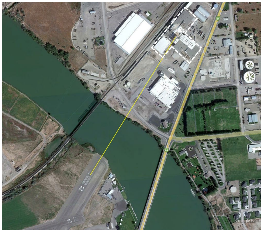
Figure 2. Zoomed in Google Earth image showing the extended centerline of the runway 20 approach with the Gem State processing plant outlined in white.
