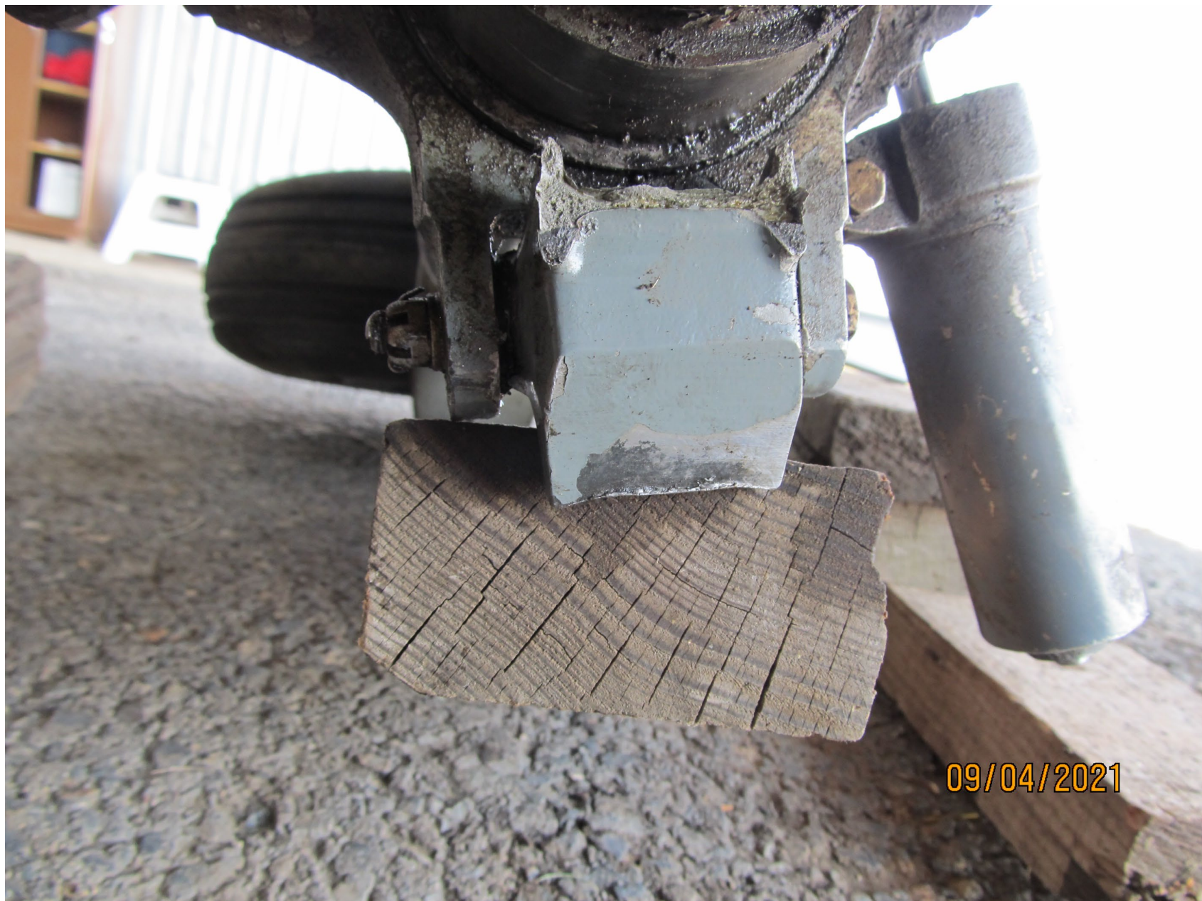
Photo 3 – Upper section of the nose gear upper torque link. Photo courtesy of the pilot.
