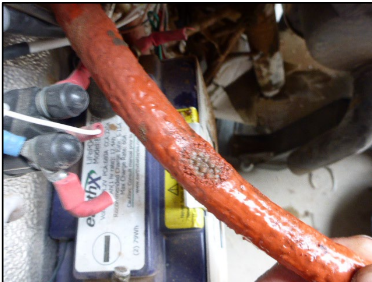
Figure 3: Oil line damaged by resting against exhaust manifold.
