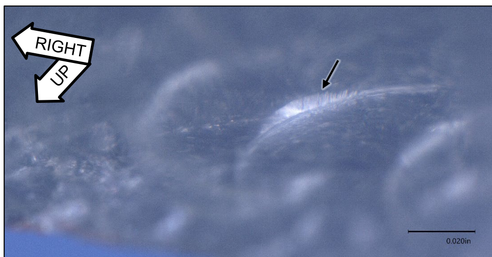
Figure 19. Crack emanating from an elliptical scratch on the exterior surface in the bond area near the origin.
