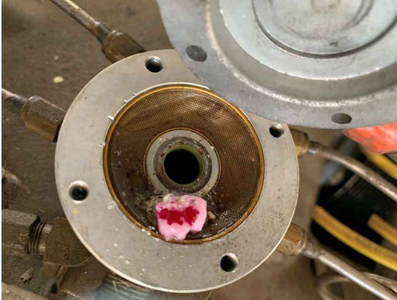
Figure 2: View of the fuel manifold valve, with water finding paste.
