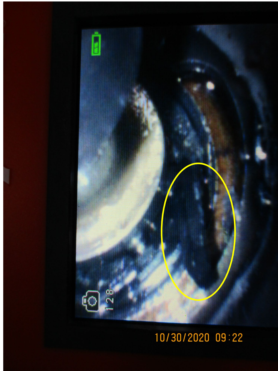
Photo 3 - View of mechanical hydraulic pump seal damage (photo courtesy of the FAA)
