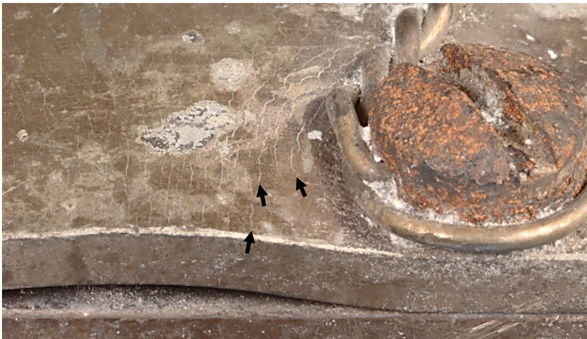
Appendix 2C. Views of the outer face of the deformed cover for the sequence valve showing micro-cracks in the oxide layer (areas indicated by black arrows).
