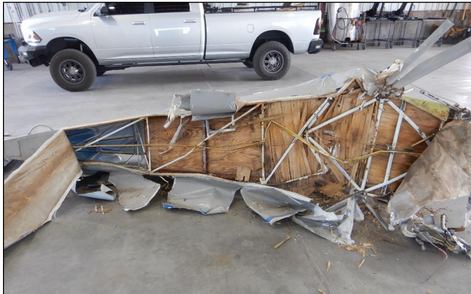
Figure 3-Lower side of fuselage with the fabric removed.
