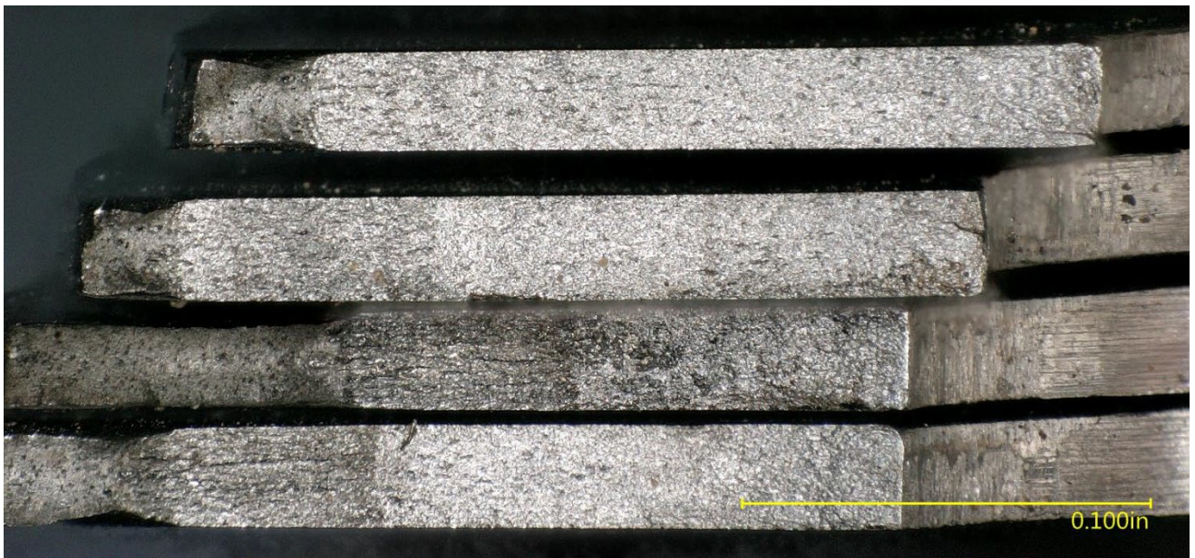
Figure 18 – Closer view of several of the TT strap fracture, showing faint crack arrest marks emanating from the bushing bore.
