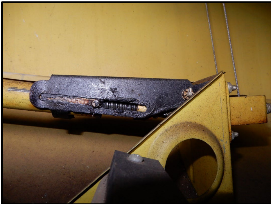
Photo 21. Elevator trim jackscrew.
