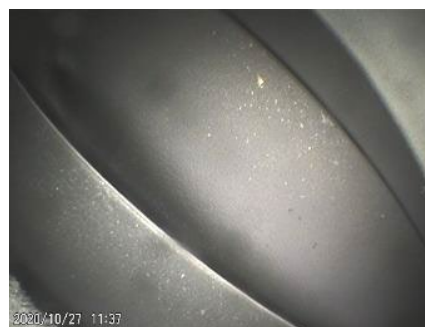
Photo 27. Metal spray on 2nd stage power turbine nozzle vanes.
