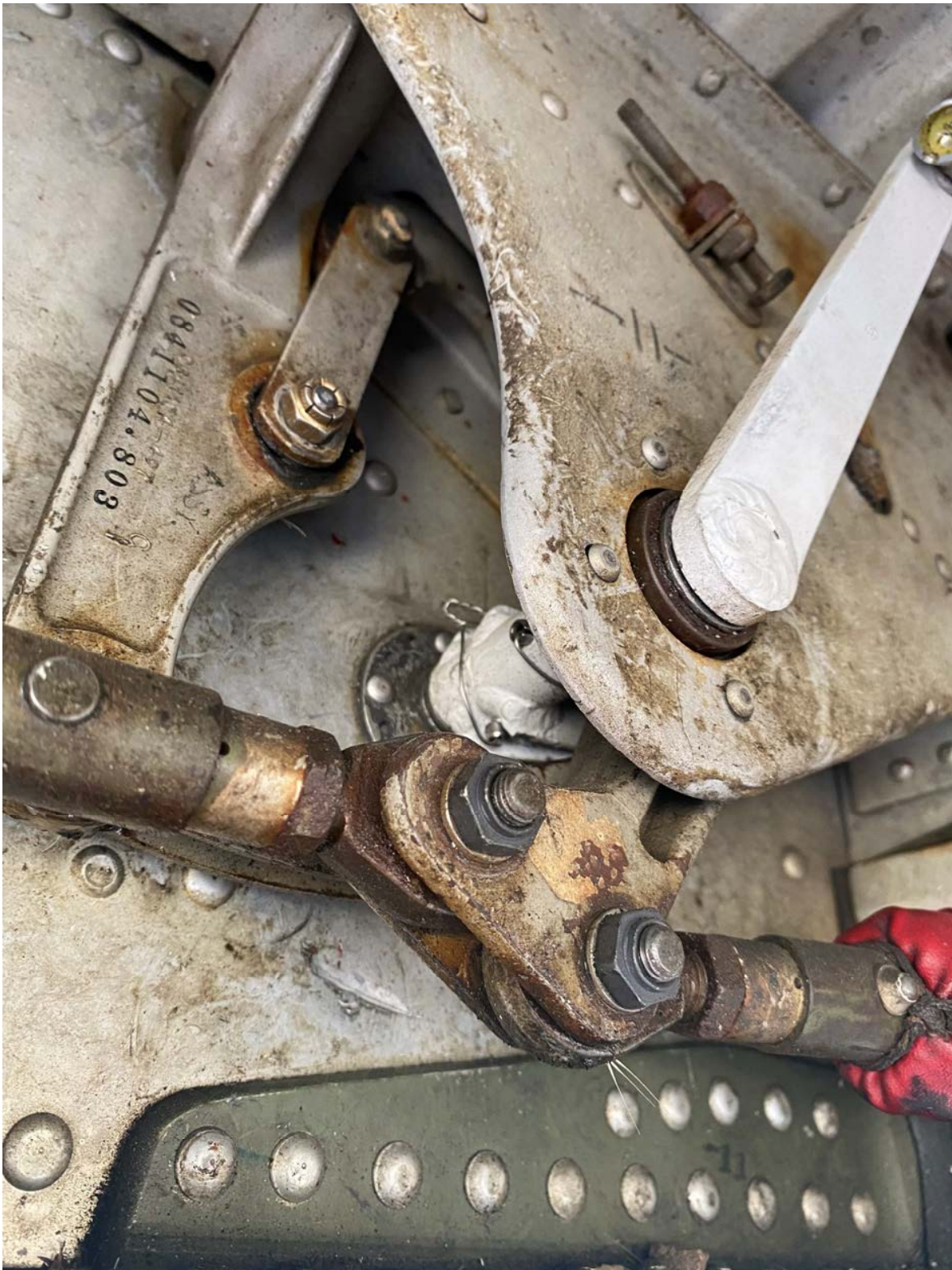
L/H Gear showing mechanism binding in as found condition
