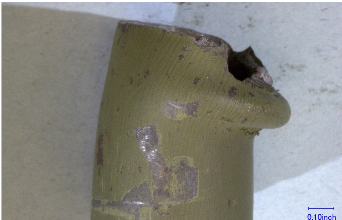
Figure 6 – View of the outboard tube fracture surface from the side.
