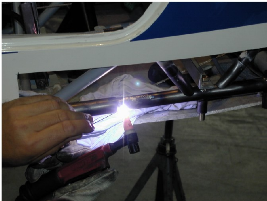
Figure 11: detail A, welded as drawn in 530-SB-05000-01/ 02 Sht2
