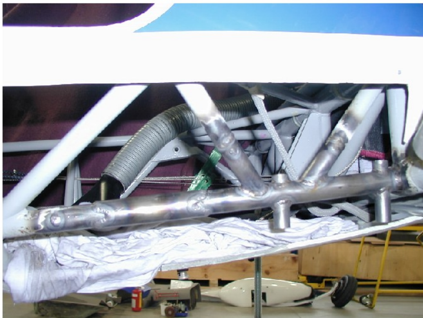
Figure 12: replaced segment (without gussets), welded
