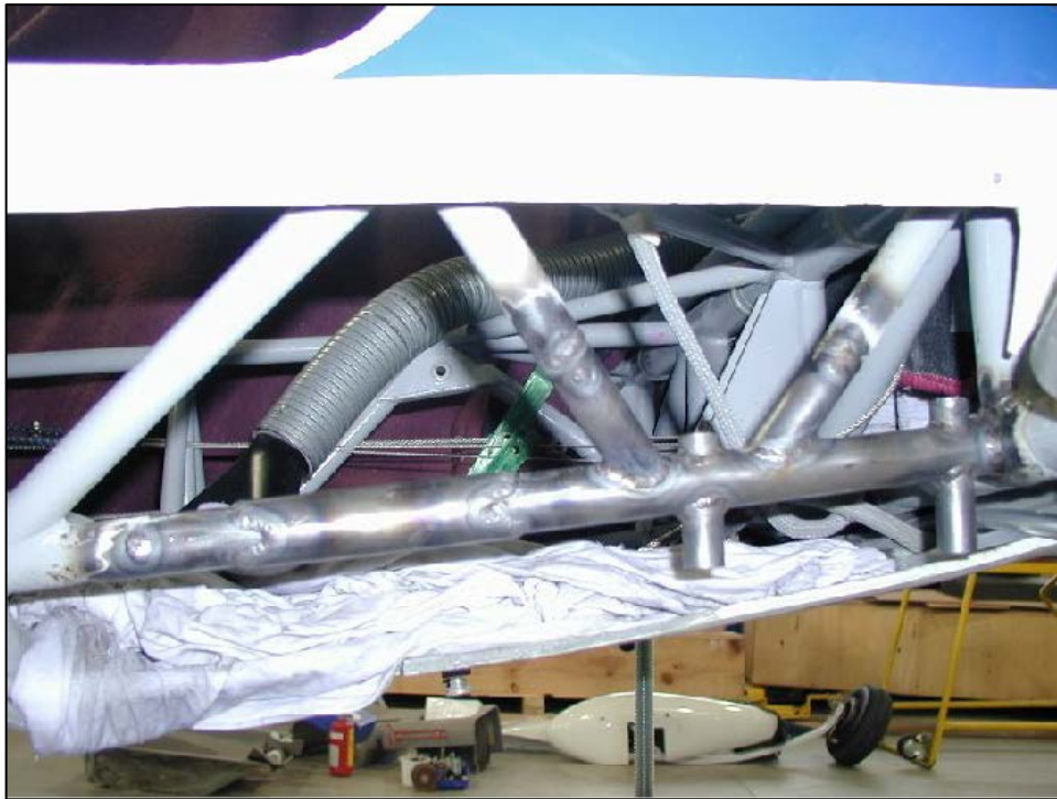
Figure 16. Image from OMF Process Specification PS-OMF 100-0006 showing the frame repair on the left side of the exemplar airplane after the replacement pieces are welded into place.
