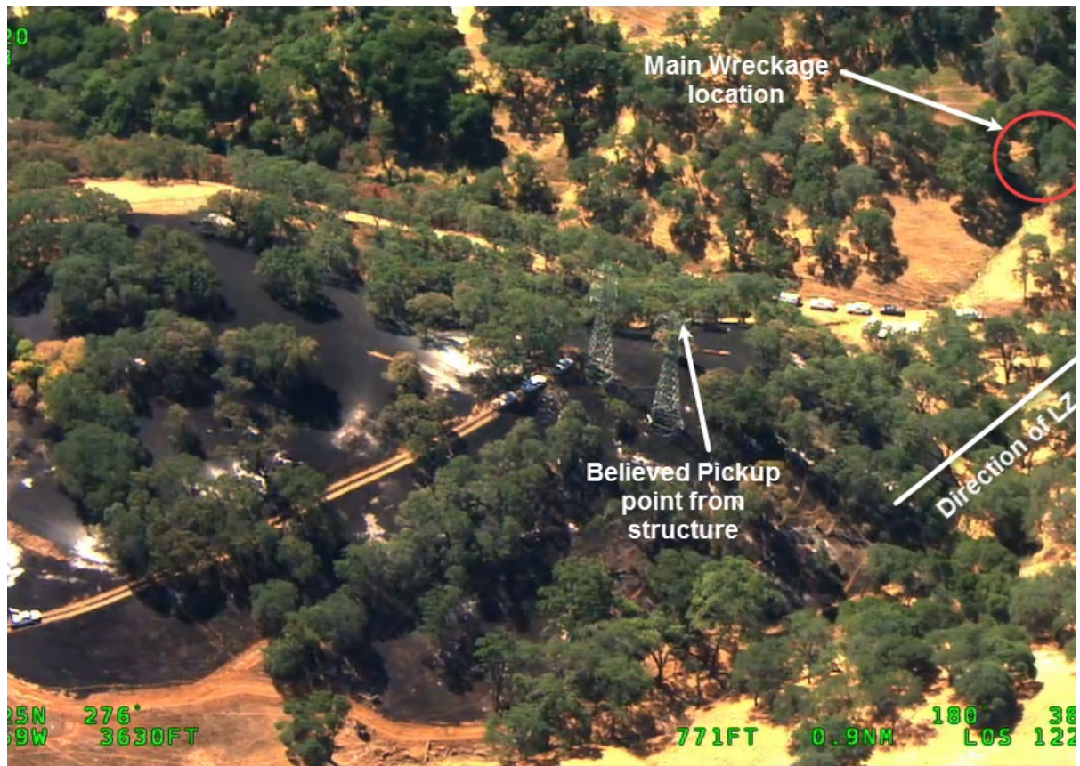
Photo 1 - Overview of Accident Site (Photo Courtesy of PGE)
