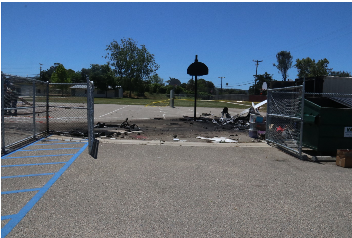
Figure 1: Overview of Accident Site
