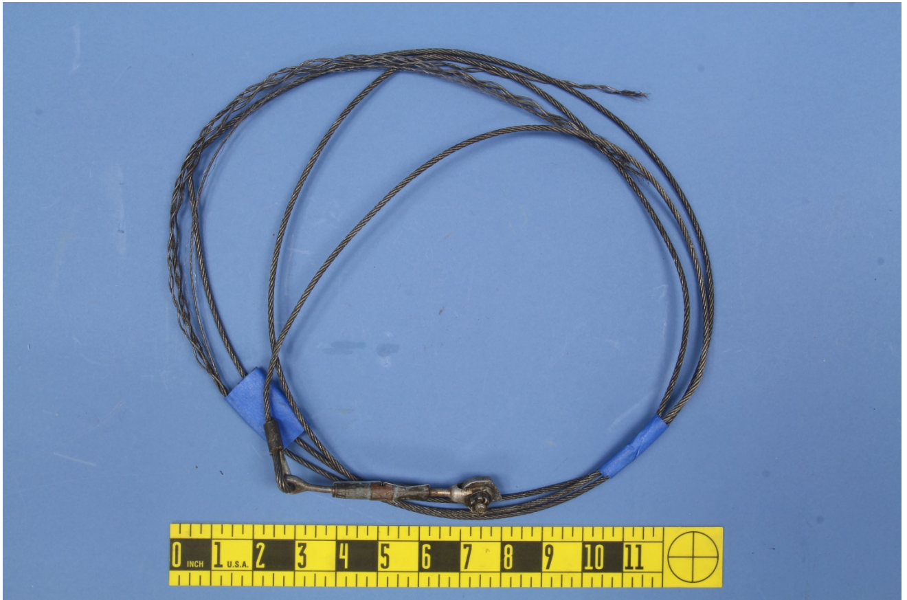
Figure 5 – The control cable remnant, as received.
