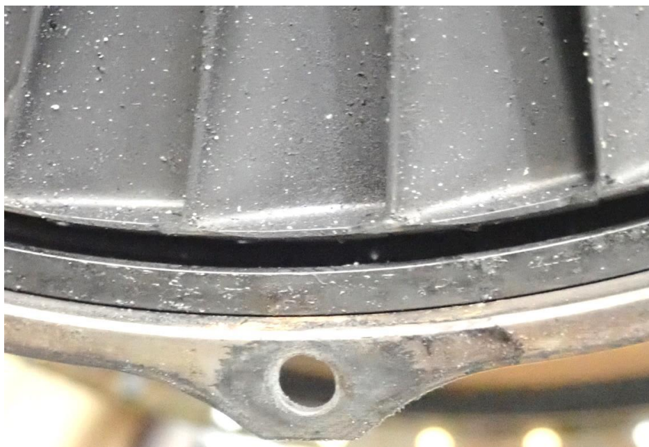
Photo No. 117, view of the upstream side
