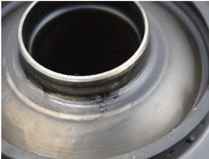
Photo No. 119, view of the upstream side
