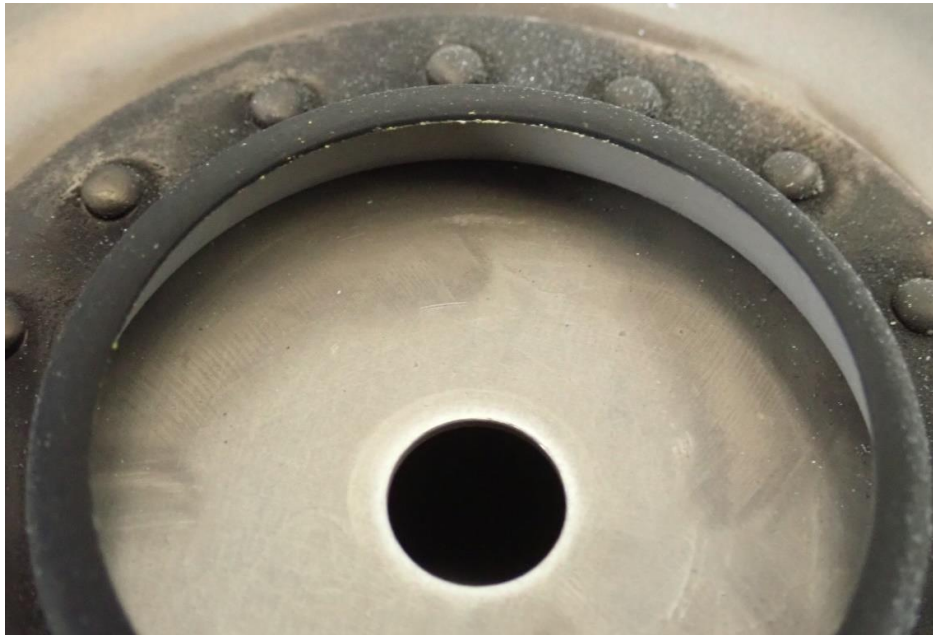
Photo No. 38, view of the upstream side
