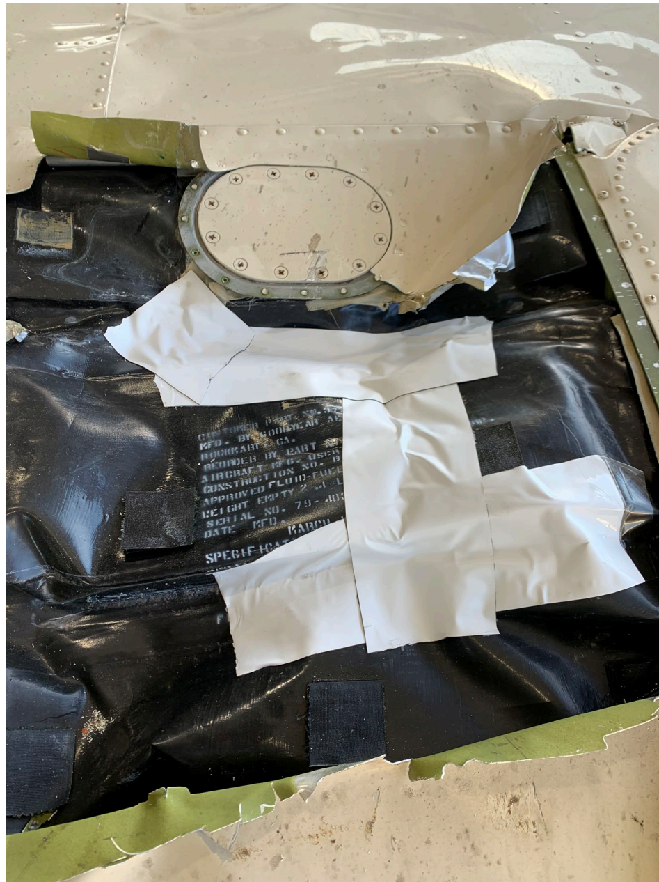
Photo 3 - View of the repair needed to fill fuel tanks with water.
