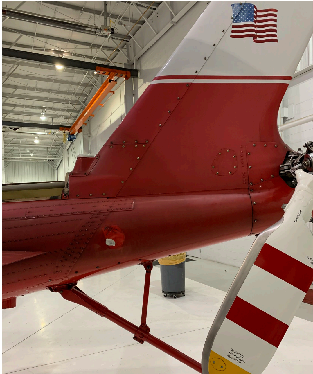
Photo 2 – Damage to Left Side Empennage (Courtesy of Intermountain)
