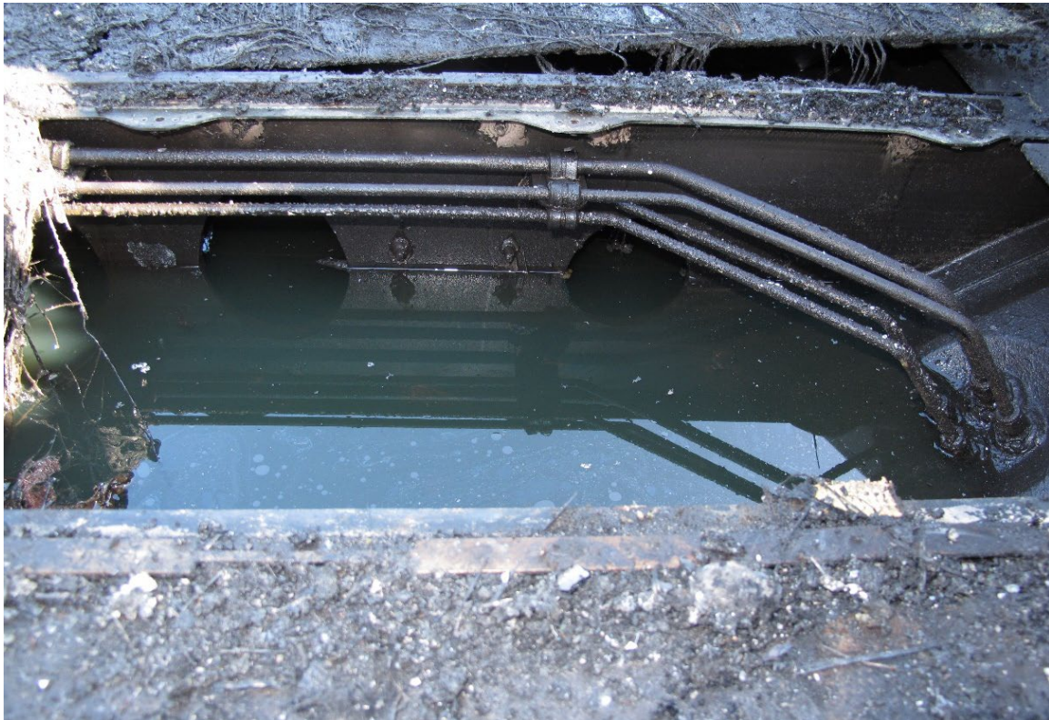
Figure 5. Close-up of hydraulic lines on left side of aircraft.
