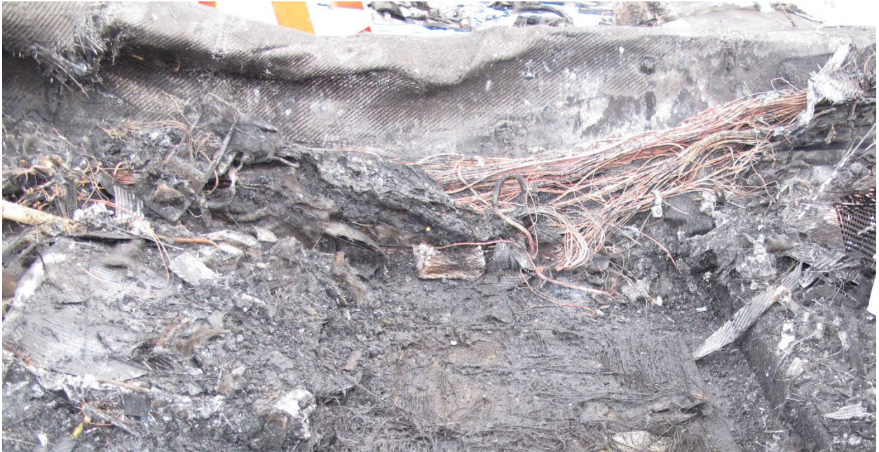
Figure 9. Section of wiring on right side wall under right egress window.
