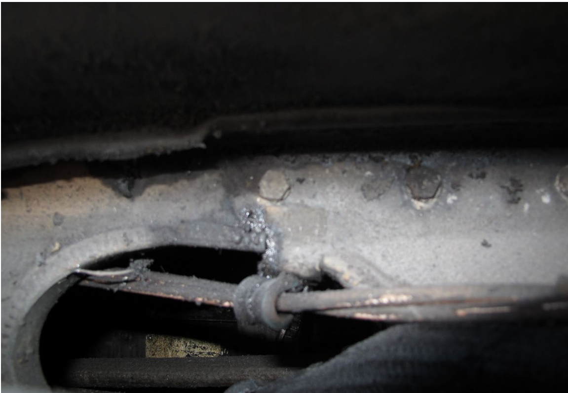
Figure 8. Close-up of underfloor wiring.
