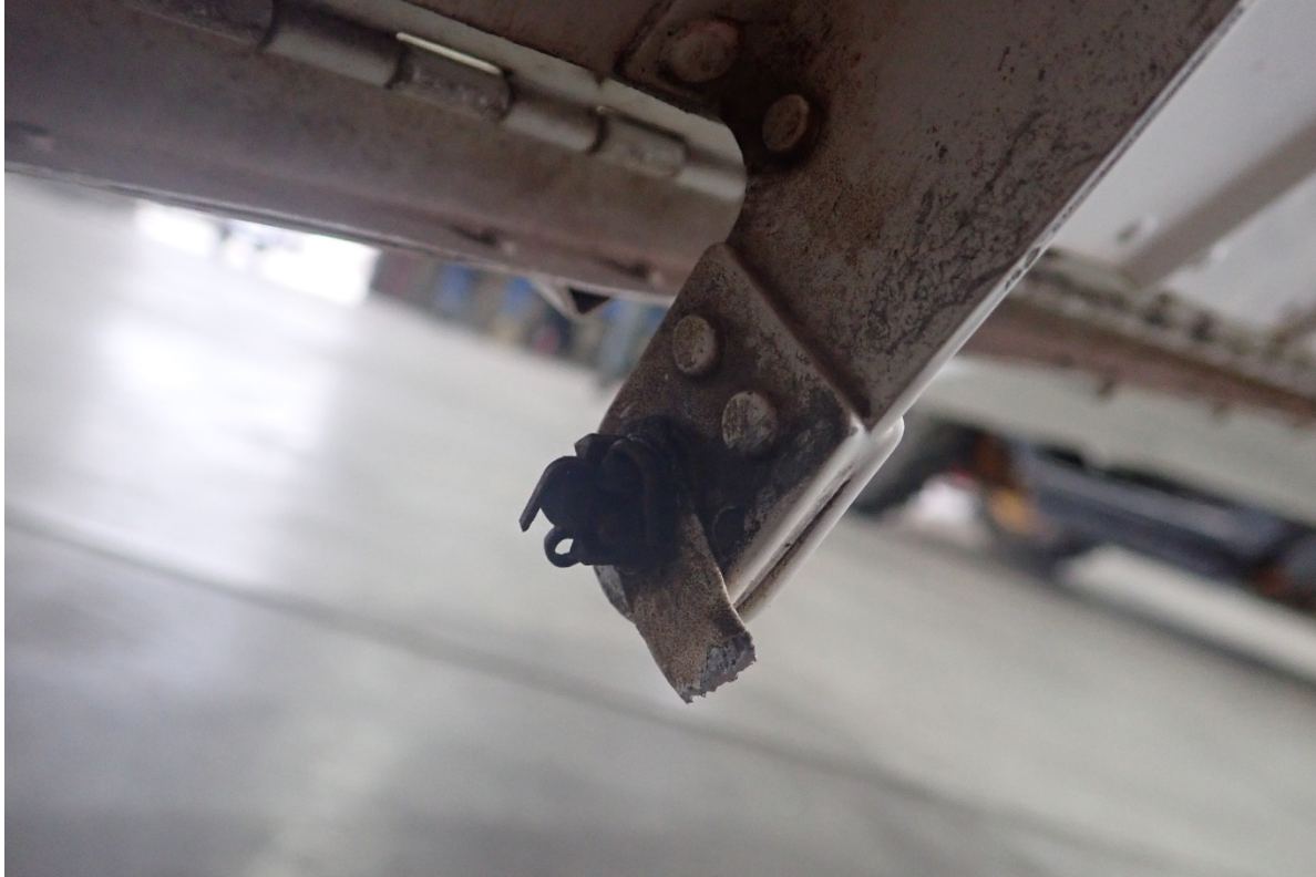
Elevator trim tab push-pull tube attach point, ASI-19-DH-079
