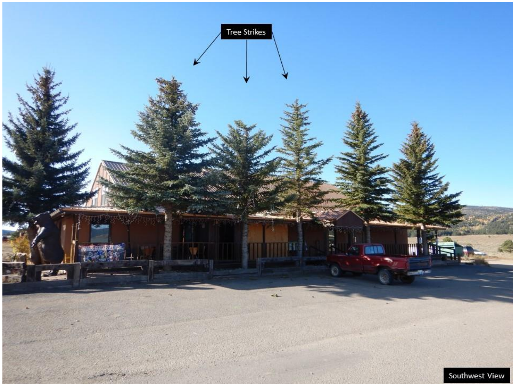
Photo 4 – Impacted trees and building.
