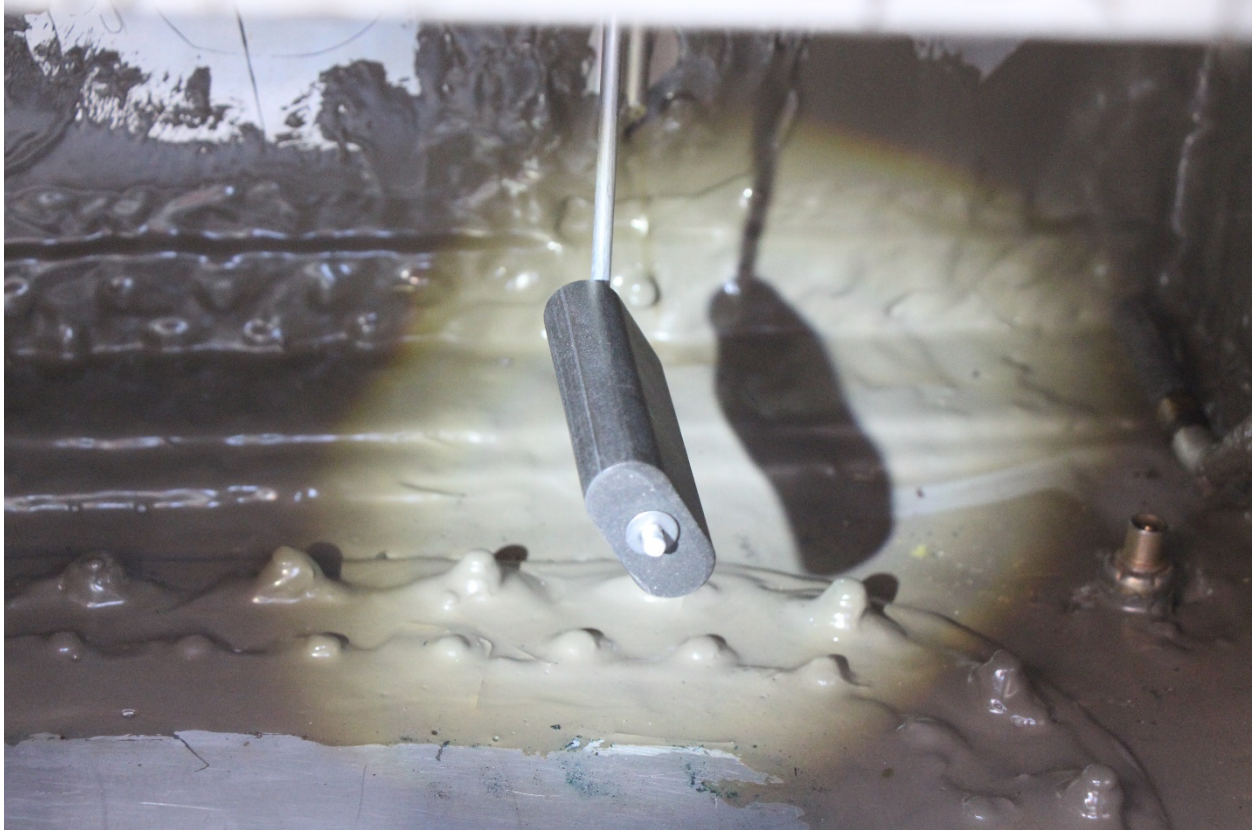
Photograph 4: Right Fuel Tank Sending Unit at Low Point In Fuel Tank
