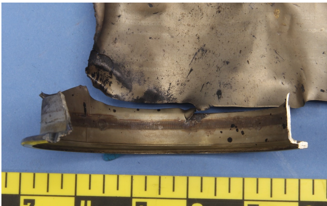
Figure 13 – View of one of the other mating flat-fracture regions of the duct remnants.
