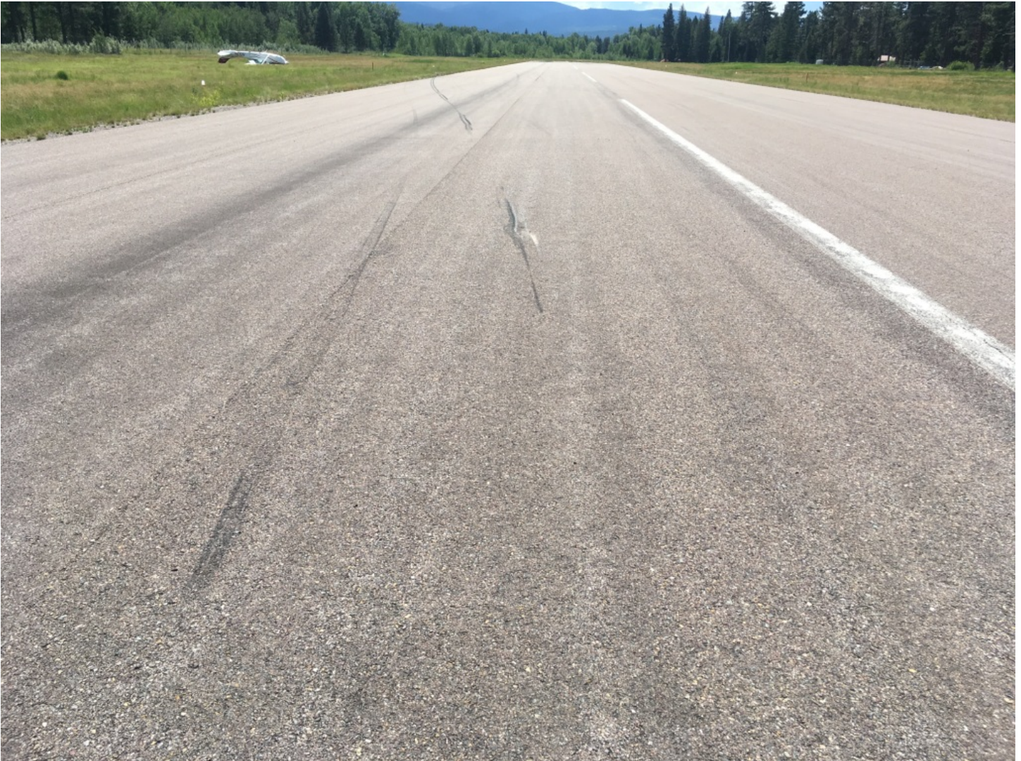
Figure 2 – Second NLG Metal Strike Scars (NOTE: Airplane moved from original at-rest location)
