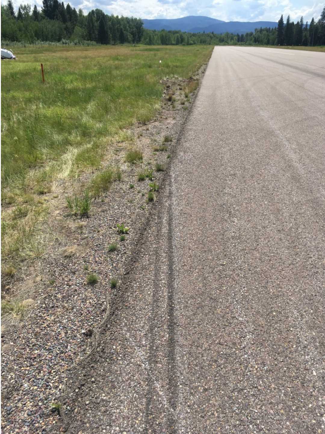
Figure 8 - NLG Exiting Runway South Edge
