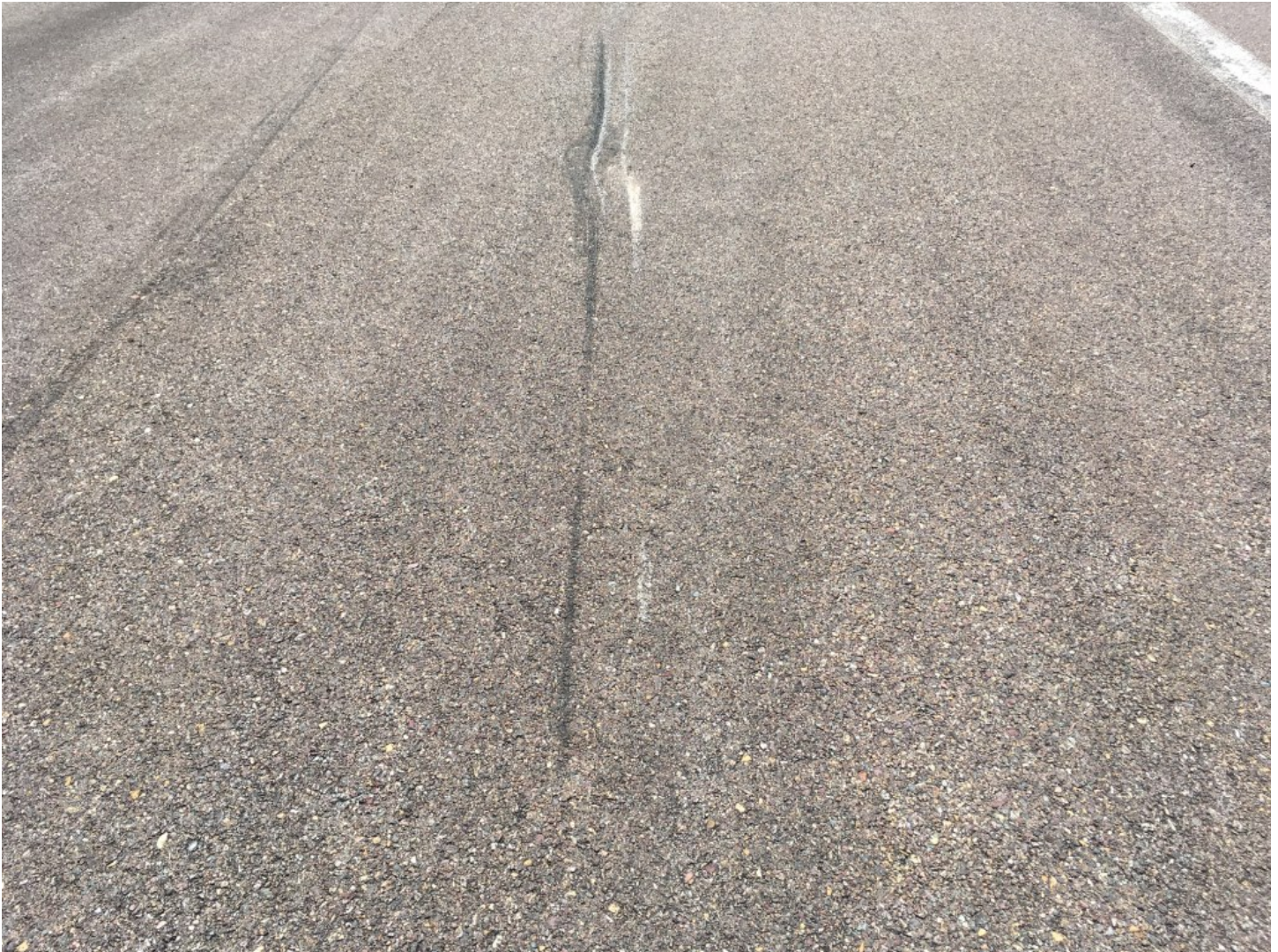
Figure 3 – Second NLG Metal Strike Scar (close up)
