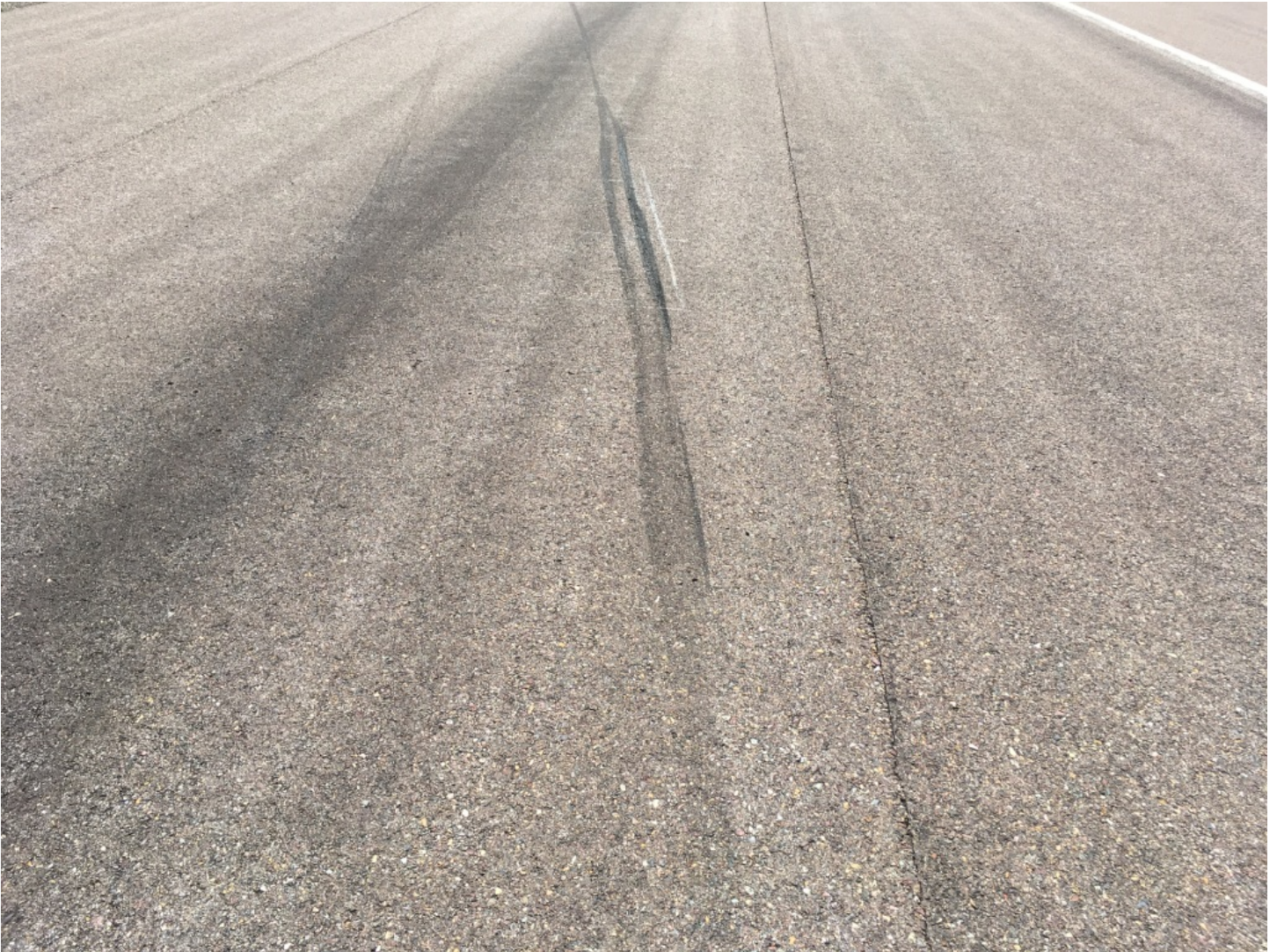
Figure 5 – Third NLG Metal Strike Scar
