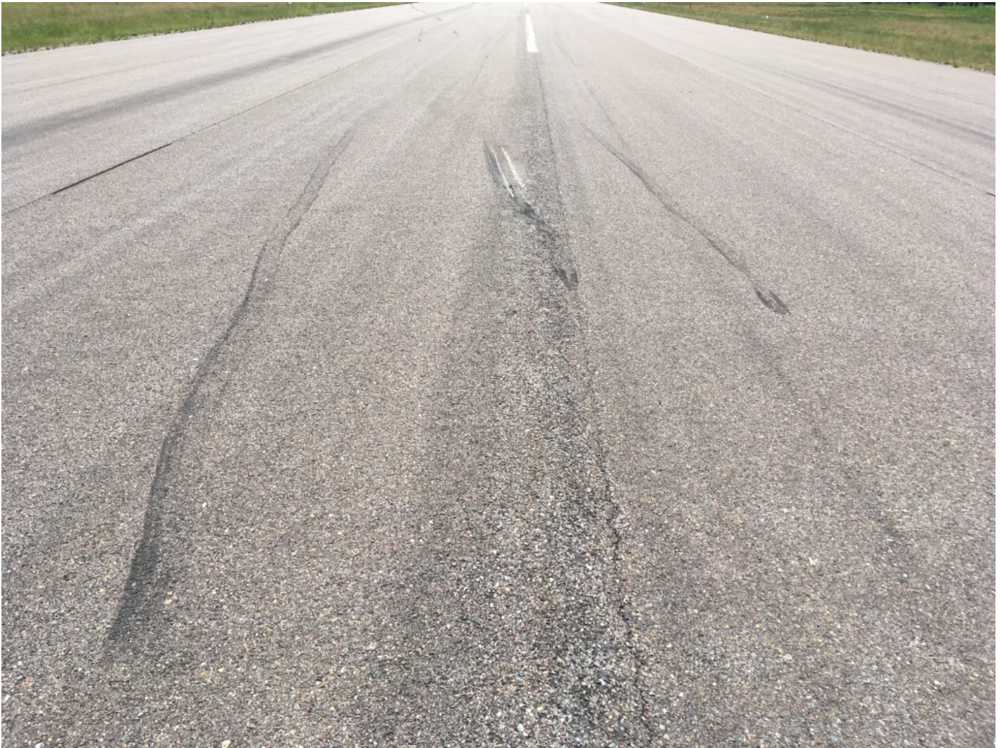
Figure 1 - First NLG Metal Strike Scars
