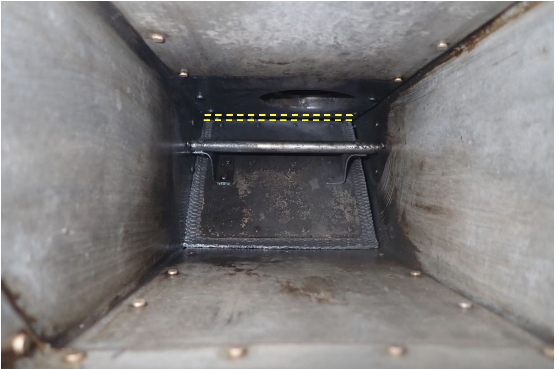
Photo 7 - Carburetor Heat Butterfly Valve with Carb in the Heat OFF Position. Viewed from Filtered Air Inlet. Missing Seal Highlighted.
