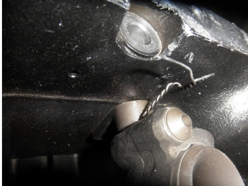
Photo No. 11: Close up view of loop of safety wire around end of boost rack.
