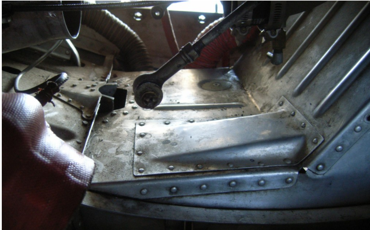
Figure 1 - Structure Below (removed) T/MA
