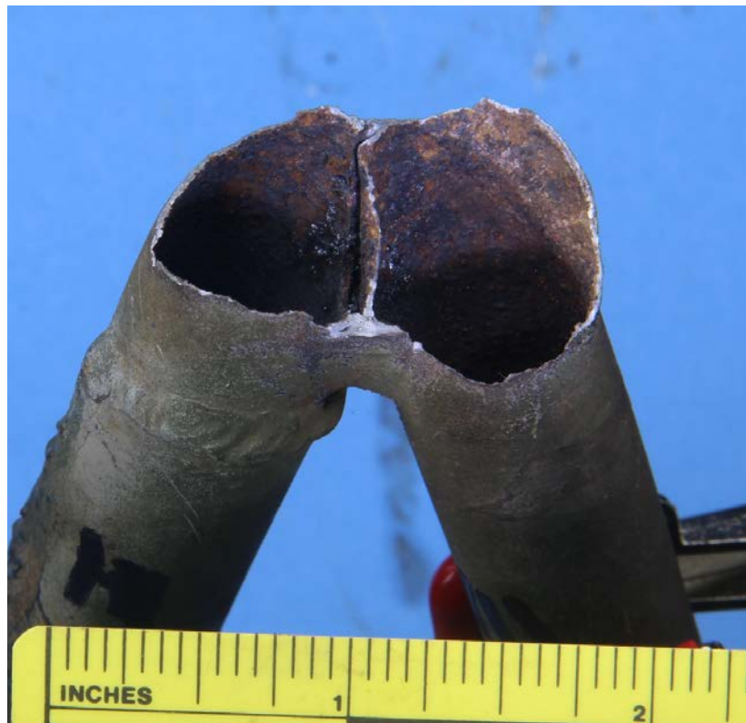
Figure 2: The top photo shows an overall view of truss tubes II and III. The white arrow points to the viewing perspective in the close-up shown in the bottom photo.
