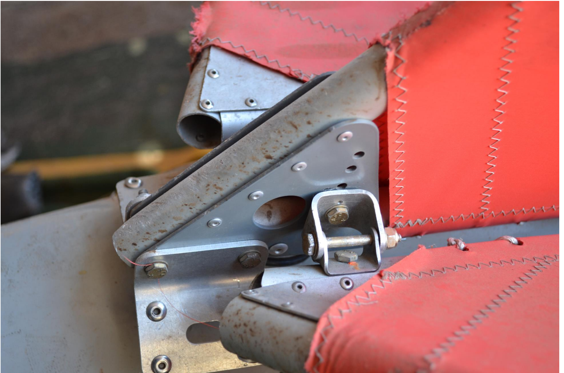
Photo 8 – Horizontal Stabilizer Forward Attachment
