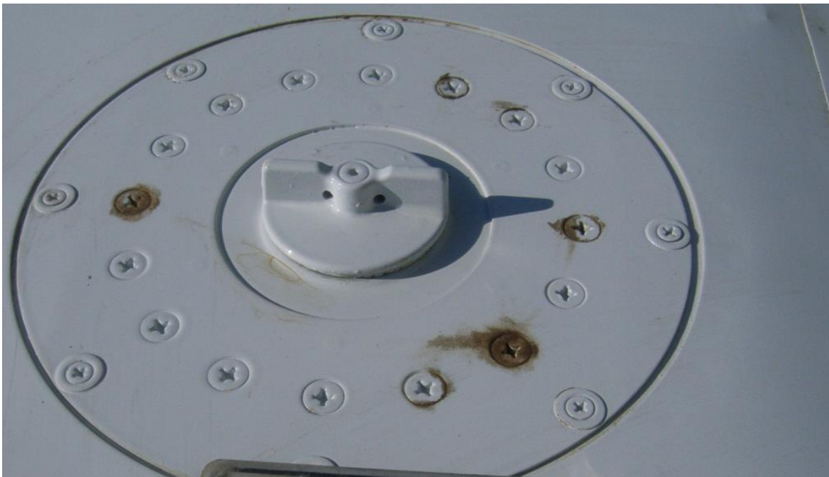
Figure 8 - Installed Fuel Cap
