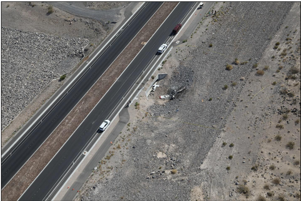
Figure 1-Accident site, aerial view (Courtesy of the Henderson Police Department)
