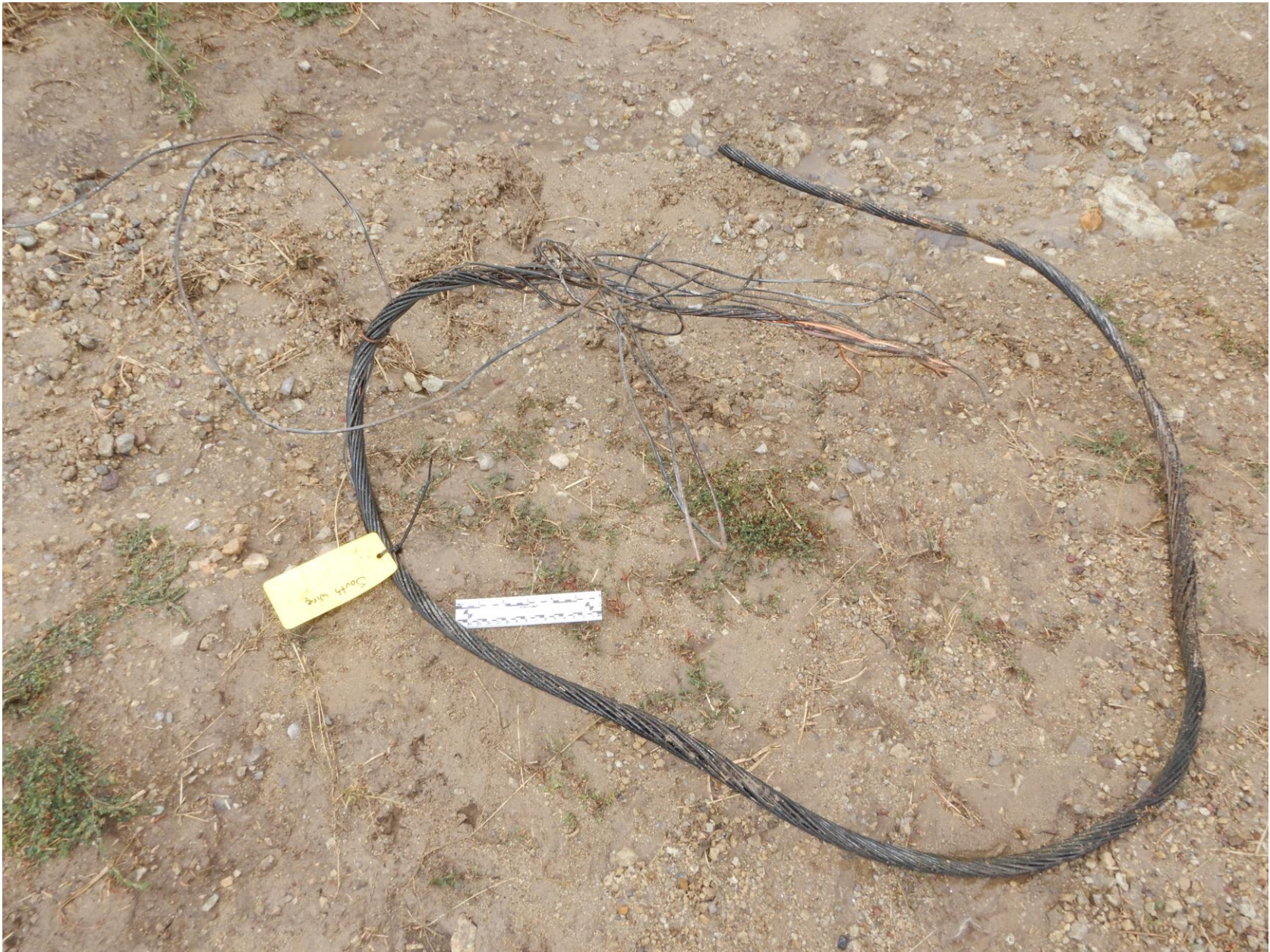
Photo 14. Eastern most power distribution line, south side
