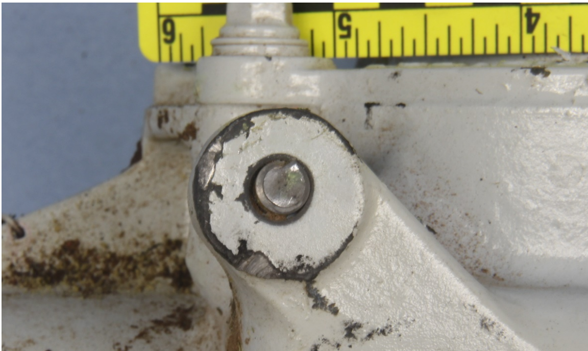
Figure 36 – Closer view of one of the fractured bolts in Figure 35.
