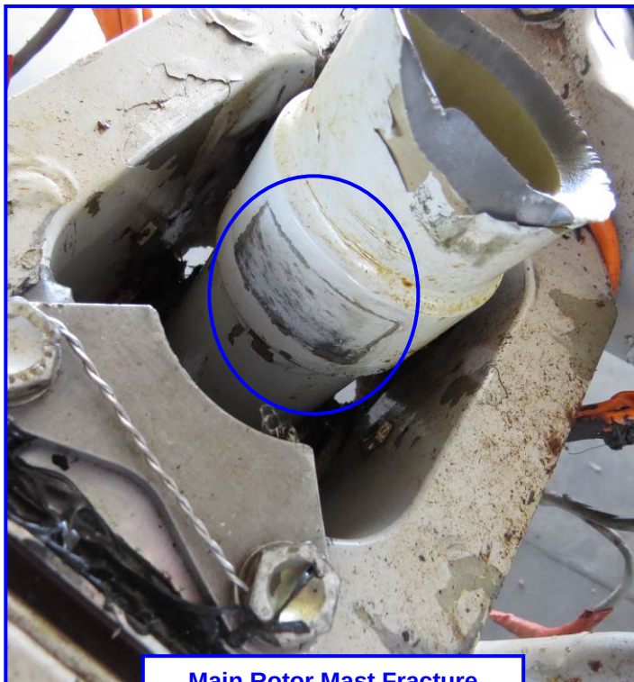
Main Rotor Mast Fracture
