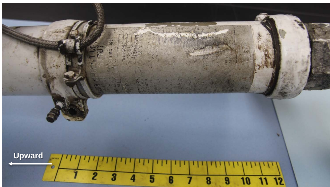
Figure 2 – The label on the landing gear strut cylinder outboard side, showing the damage to the text.
