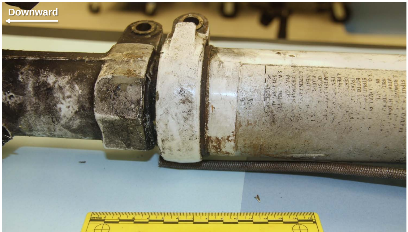
Figure 7 – View of the loose joint on the strut cylinder from the outboard surface, after removal of the linkage and connecting bolt assemblies.
