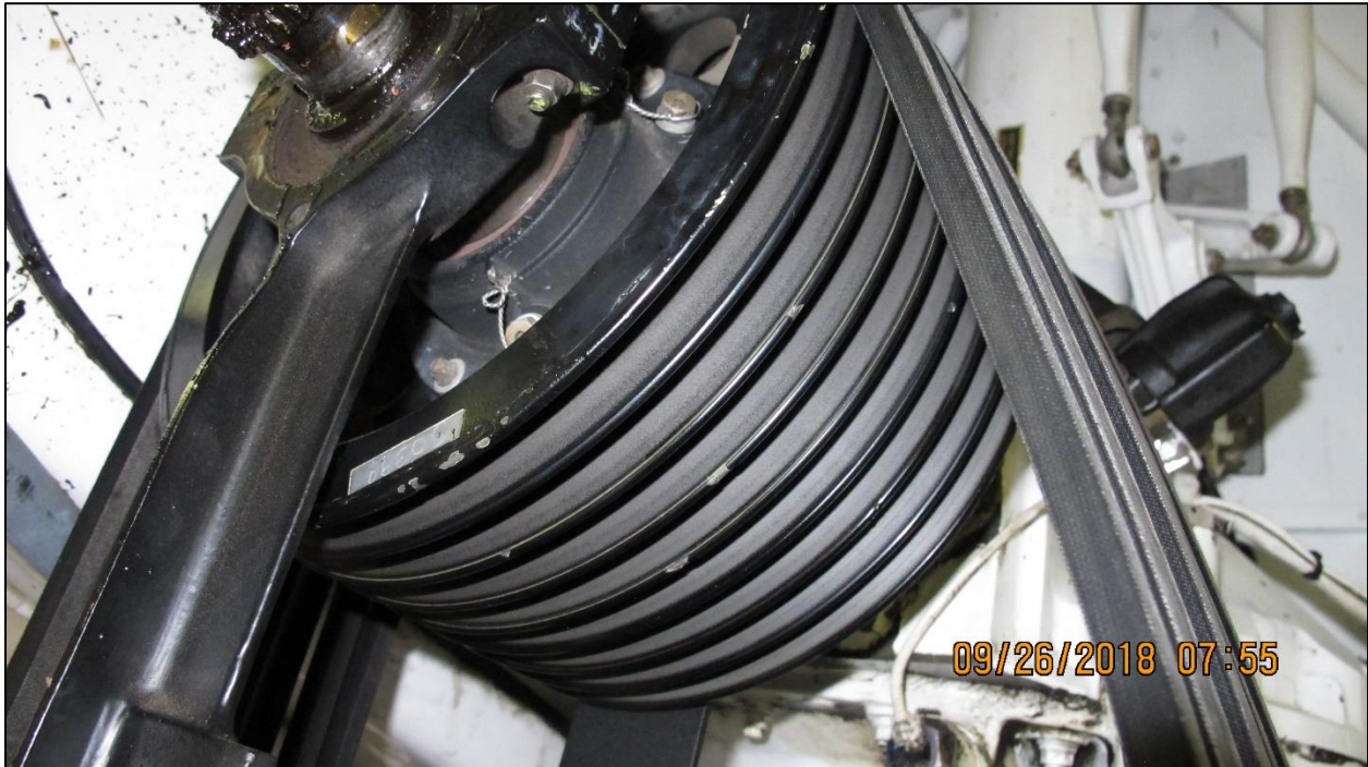
Figure 6-Drive Belts and Belt Sheave
