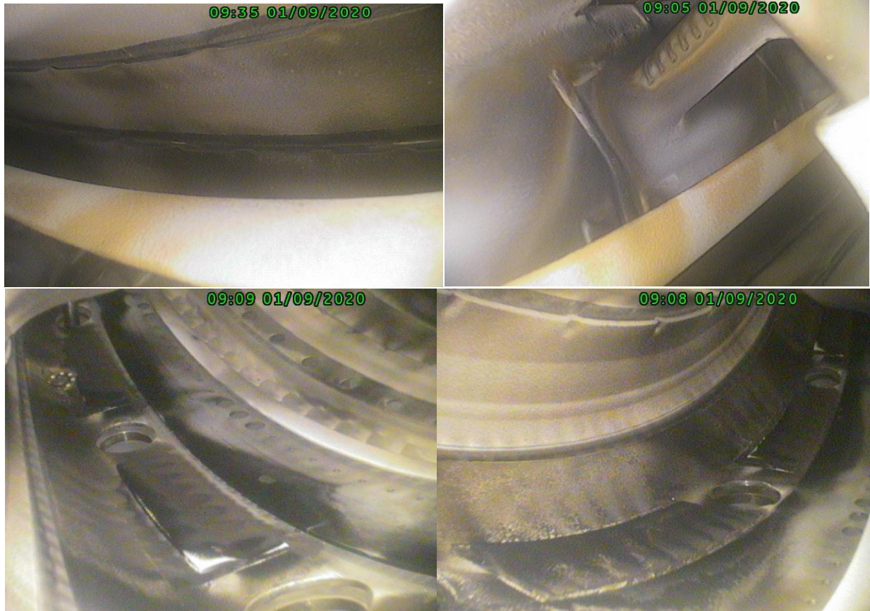
Photo No. 3 Combustion chamber area
