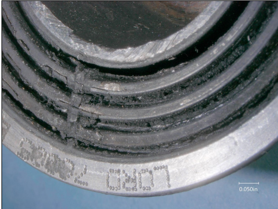
Figure 15. Close view of the radially outward side of the removed inboard teeter bearing.
