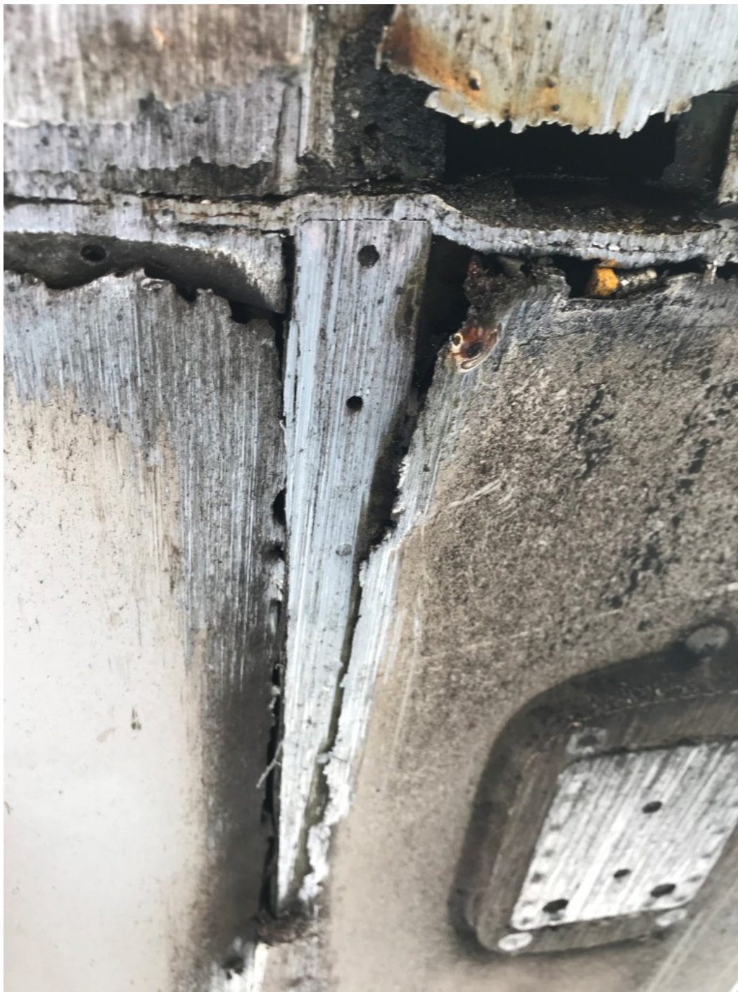
Figure 6 - Fuselage Lower Skin Damage
