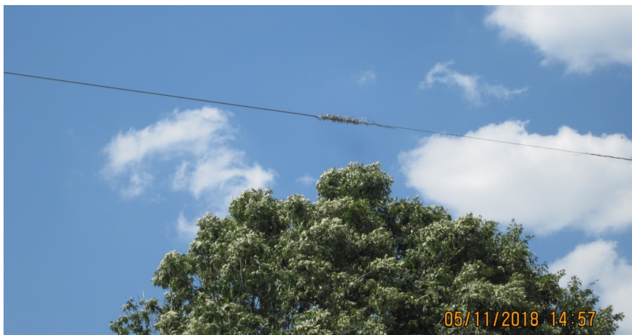
Figure 2 - Struck Tree and Struck Powerline
