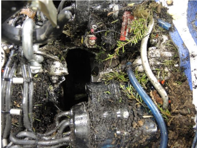
Hole in crankcase between cylinders 1 and 2
