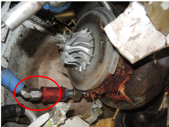
The turbocharger oil drain line from the check valve to scavenge pump was found hand tight at the check valve connection (circled above).
